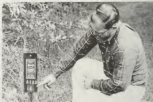
Markers indicate where the cable is!
