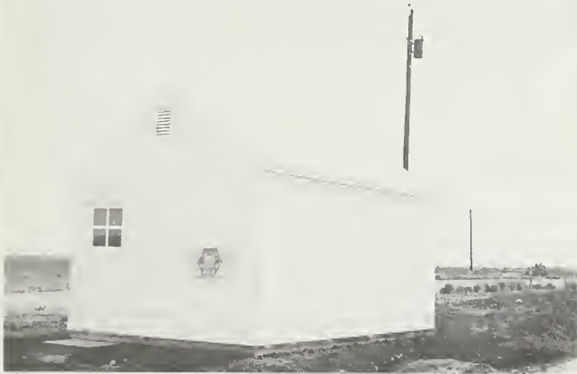
Early unattended dial offices could be quickly built to house basic equipment. They served as the link between subscribers' homes and the outside world.
