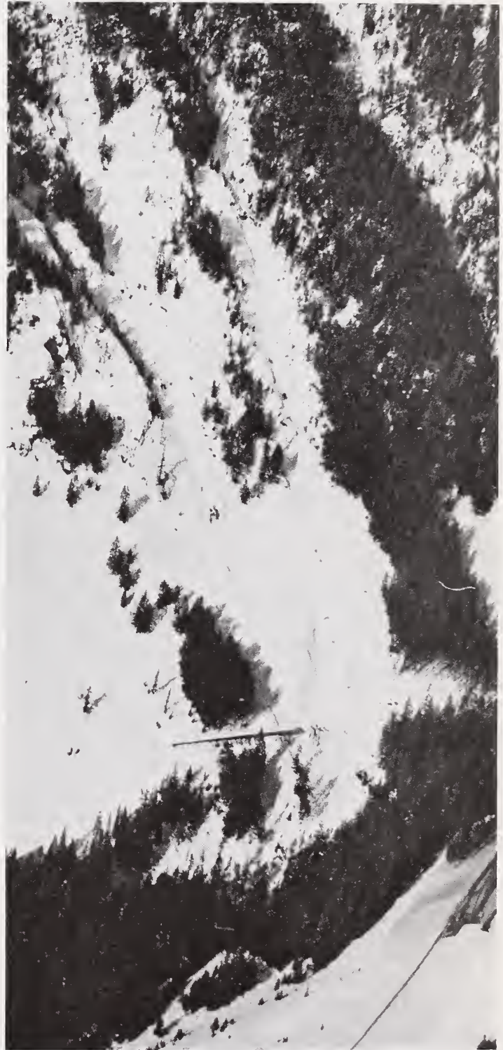
No. 71-11. Franklin Falls, Snoqualmie Pass, Washington. The highway work bridge can be seen near the foot of Denny Mountain. In this photograph, only the left-hand portion of the bridge is standing; the right-hand portion was destroyed by the avalanche. The existing route I-90 can be seen in the lower right foreground.
