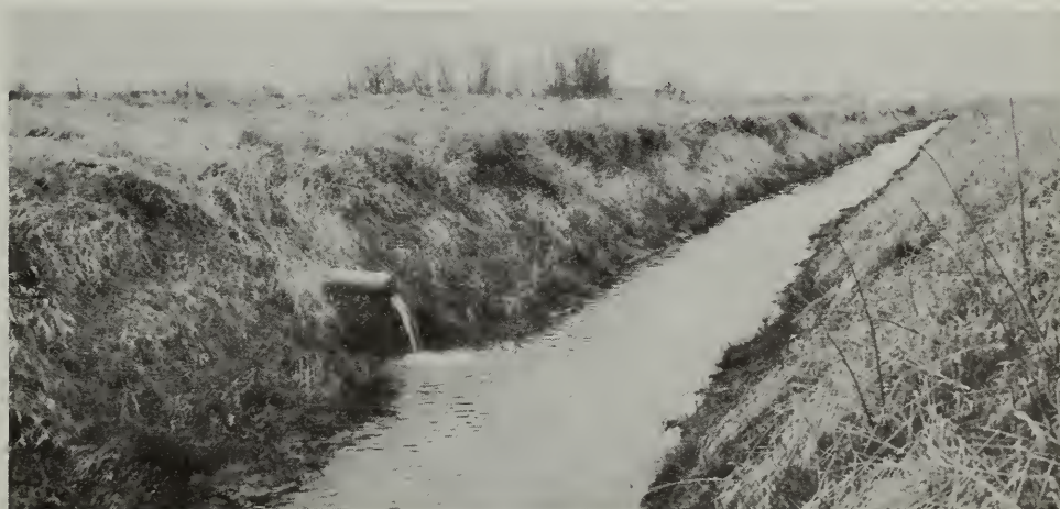
An outlet ditch with proper depth and capacity.
