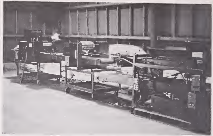
Figure 7-3.—Integrated hopper, filler, and tamper for containers.
