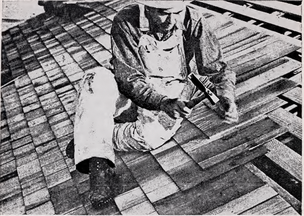
Figure 1.—Laying wood shingles over slats.
