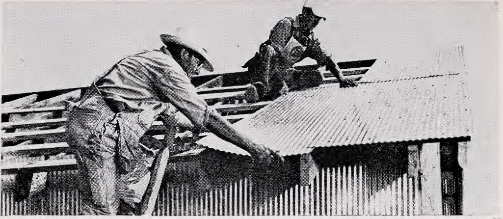
Figure 11. —Laying corrugated galvanized-steel sheets.
