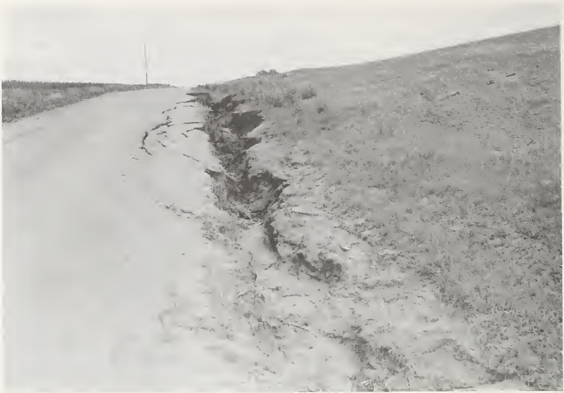
Photo 9 - Typical gully erosion undercutting a blacktop road
