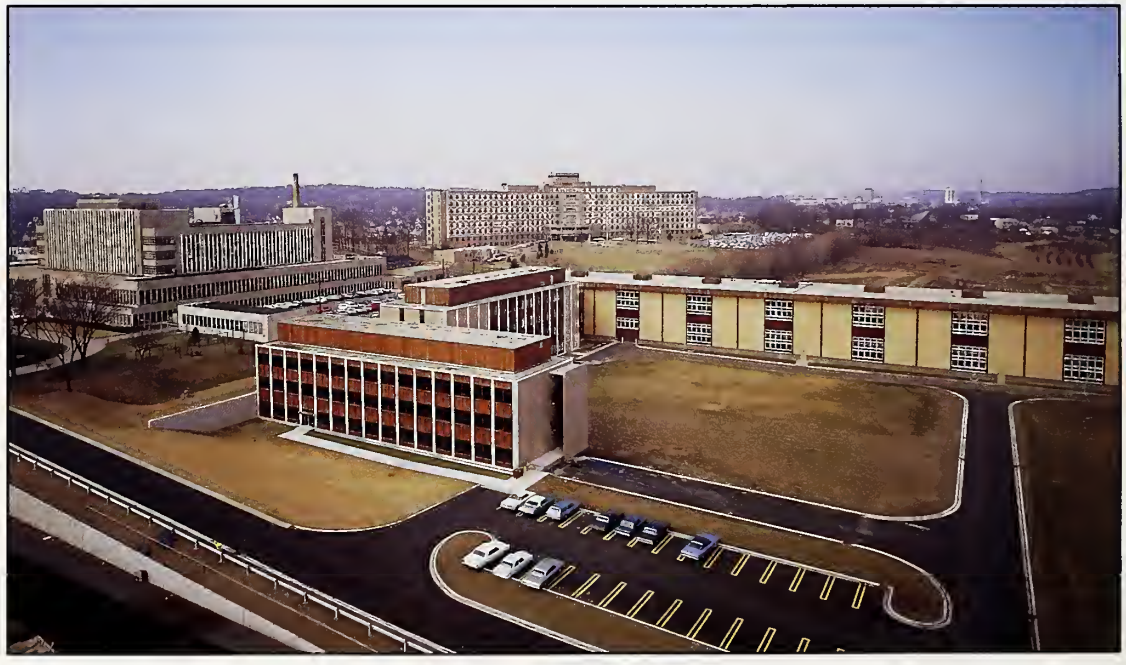
The Forest Products Laboratory comprises 10 buildings on 22 acres. Most of the pulp and paper facilities are located in a single building (right).
