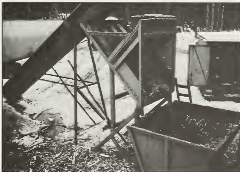
Figure 10—The magnet-conveyor system.
