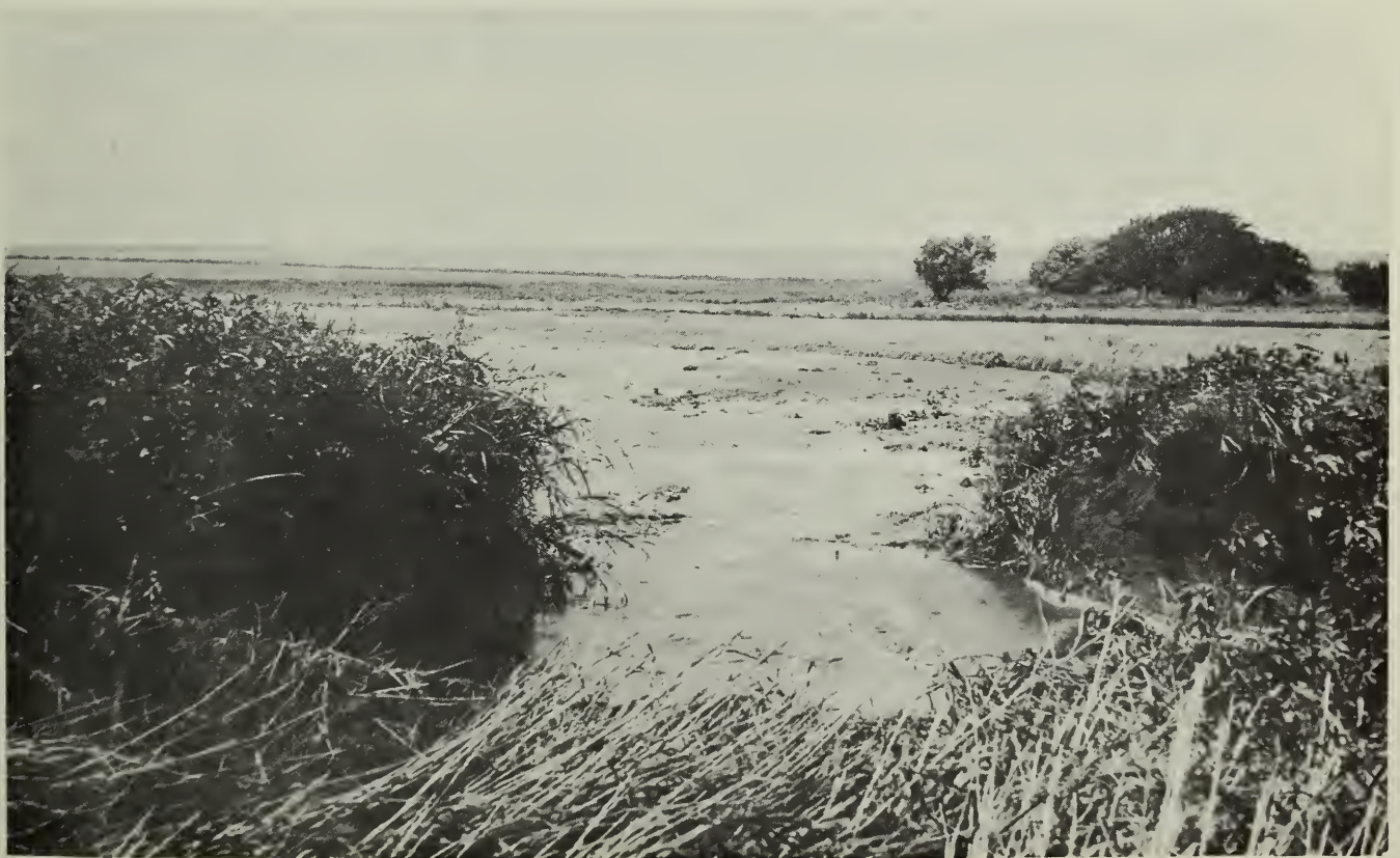
Levee and Sediment Damage - Storm of June 1963
