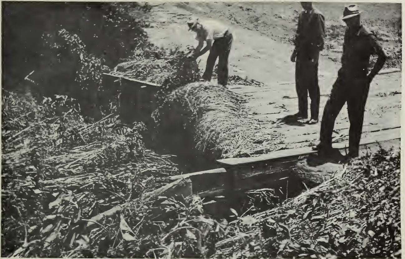
Road and Bridge Damage - Storm of June 1963
