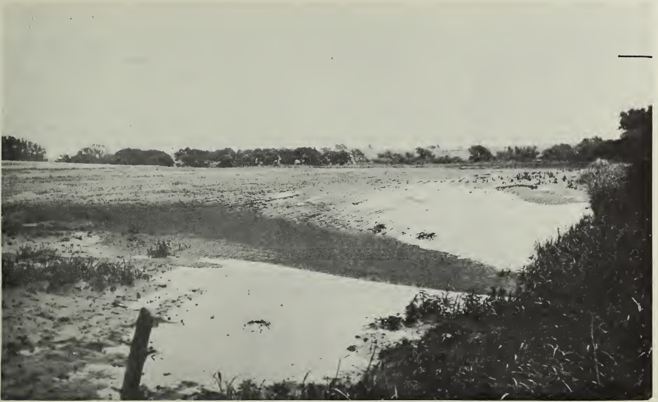
Sediment Damage - Storm of June 1963
