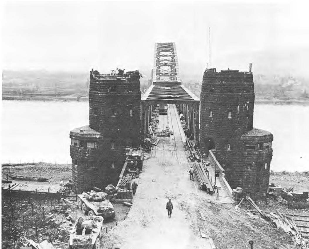
LUDENDORFF RAILROAD BRIDGE AT REMAGEN
