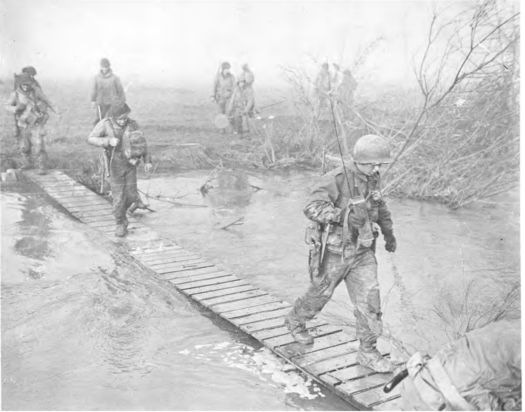
FOOTBRIDGE ACROSS THE ROER SERVES MEN OF THE 30TH DIVISION
