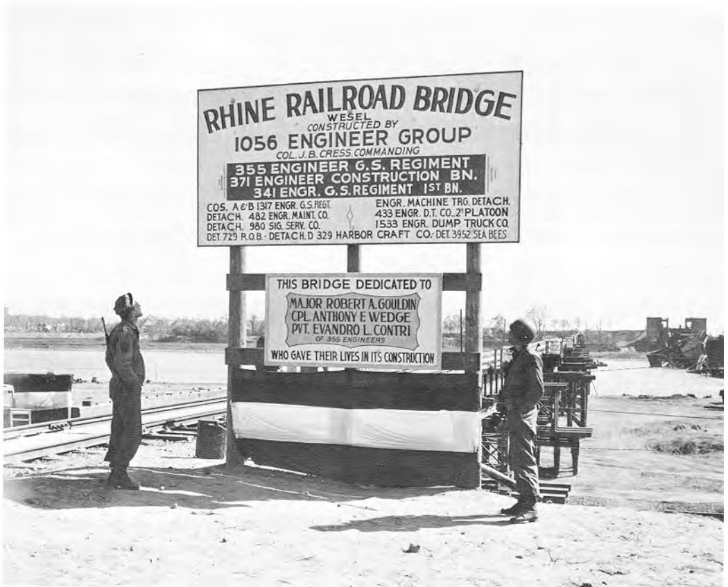
THE RHINE RAILROAD BRIDGE AT WEASEL
