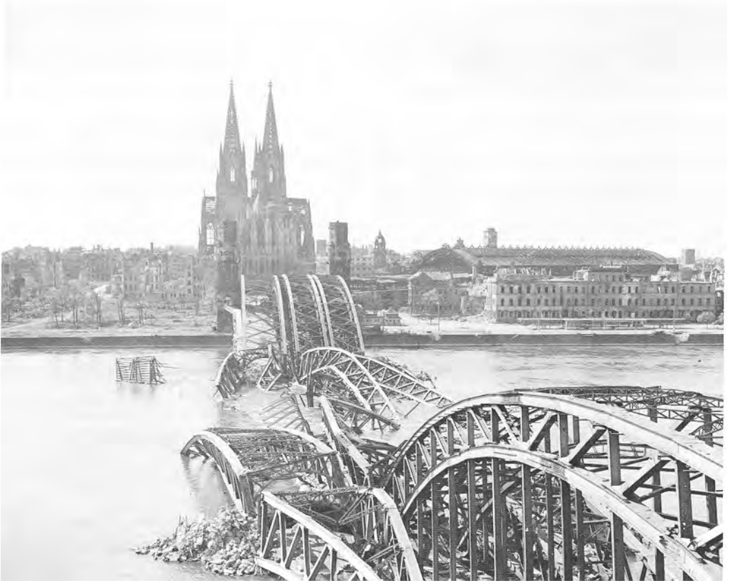
THE DEMOLISHED HOHENZOLLERN BRIDGE at Cologne with cathedral in the background.
