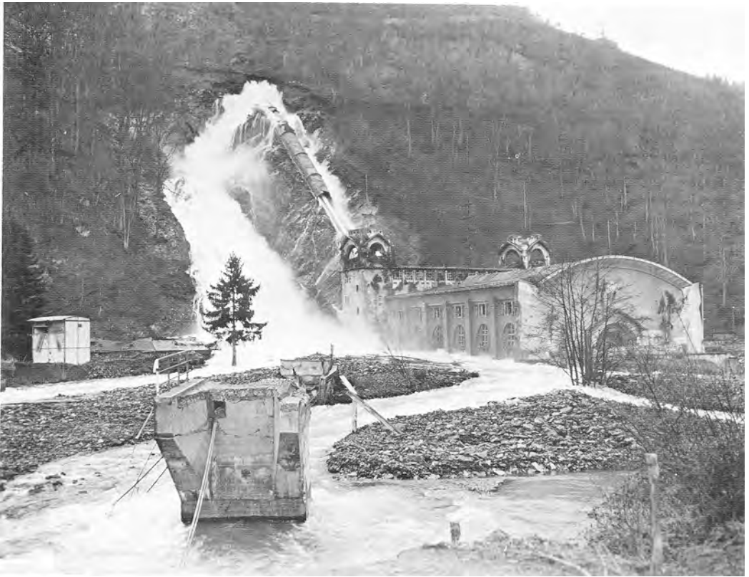
DAMAGE TO THE SCHWAMMENAUDEL DAM causes flooding of the Roer River.
