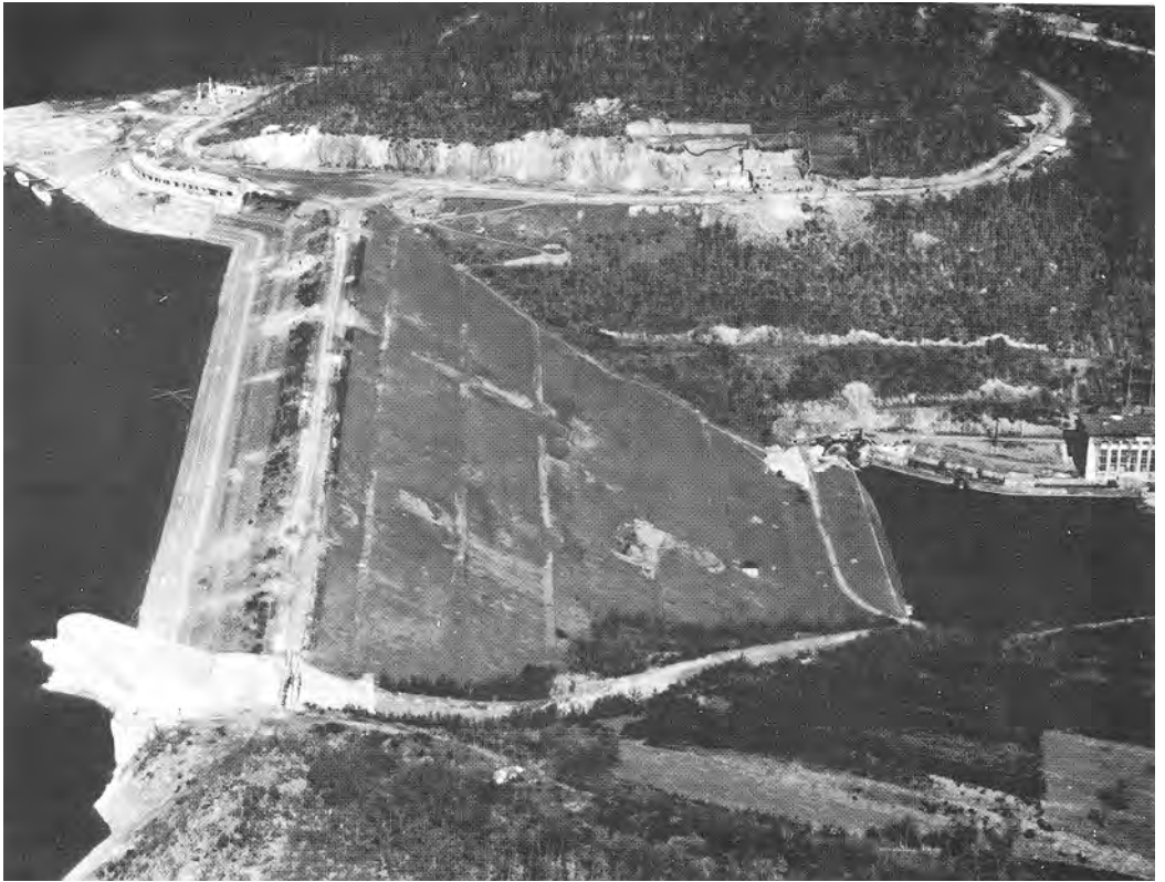
THE SCHWAMMENAUEL DAM
