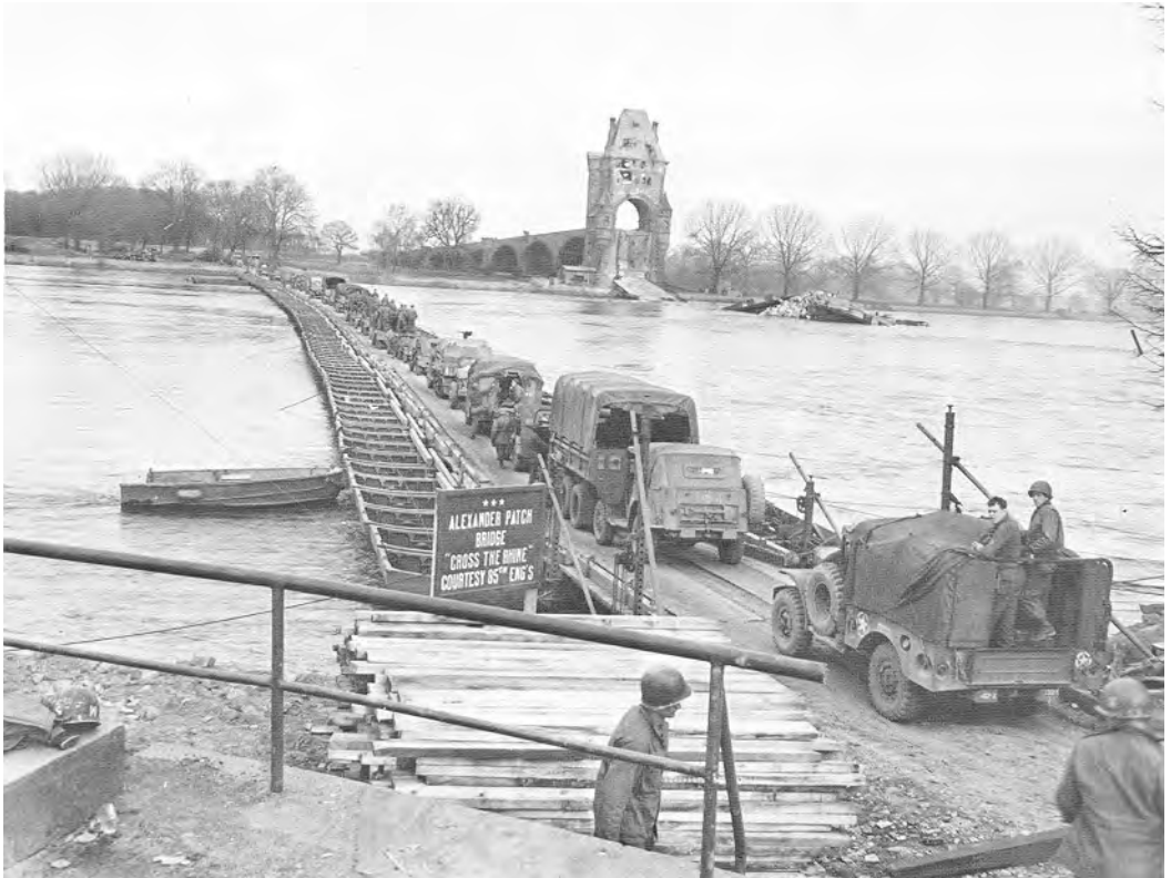
PONTON BRIDGE ACROSS THE RHINE SERVING SEVENTH ARMY
