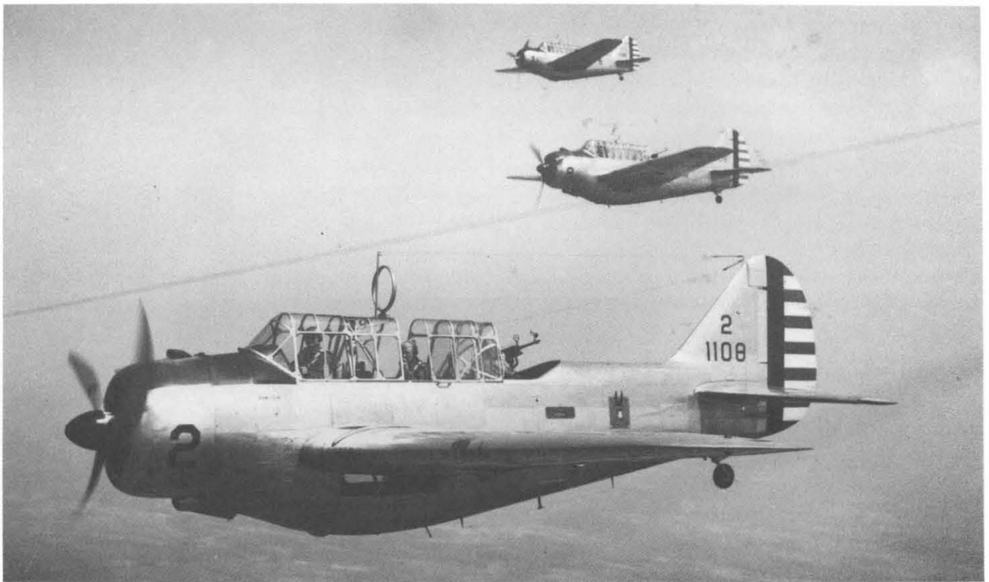
Then in the late thirties the Air Corps sought a more powerful, faster, all-metal monoplane type for observation tasks. The North American O-47 ( top ) and Curtiss O-52 ( bottom ) were excellent flyers. The O-47 had an observation bay below the wing; the O-52 used a high-wing configuration to allow the flight crew an unobstructed view below.
