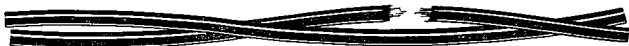
B OPEN CIRCUIT-A BREAK IN ONE OR BOTH WIRES OF A PAIR.
