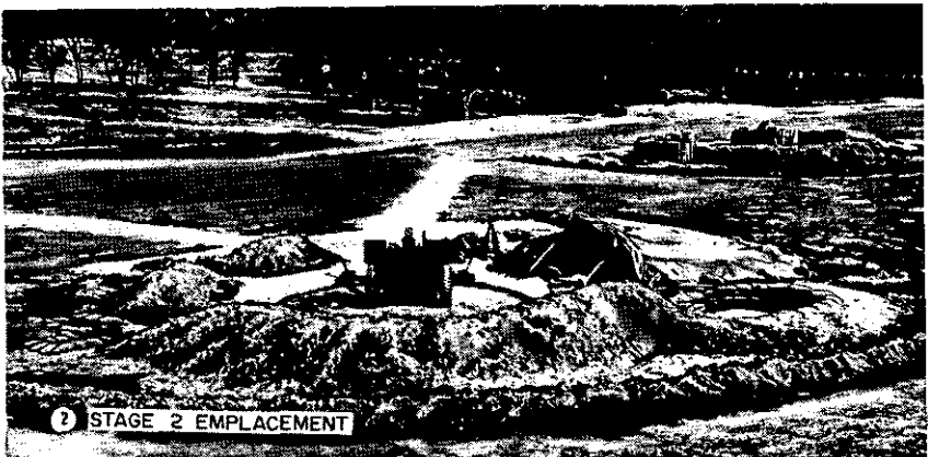
Figure 67. Progressive development of 105-mm howitzer emplacement.
