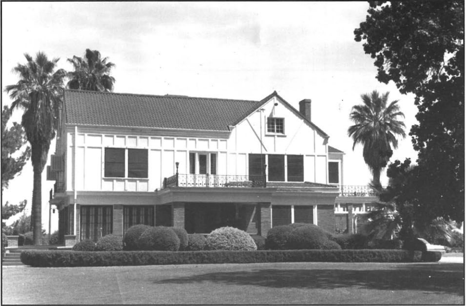
Administration building after its restoration.
