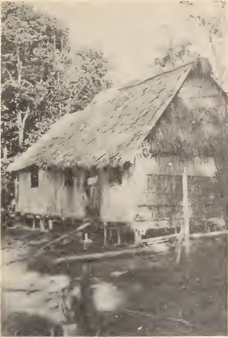
FIGURE 9.- Close-up of caboclo's hut, showing its construction and the family of the castanheiro. The house is built on piling because of dampness.
