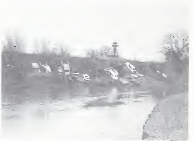
Figure 3.--Complete protection between jetties by automobile bodies.
