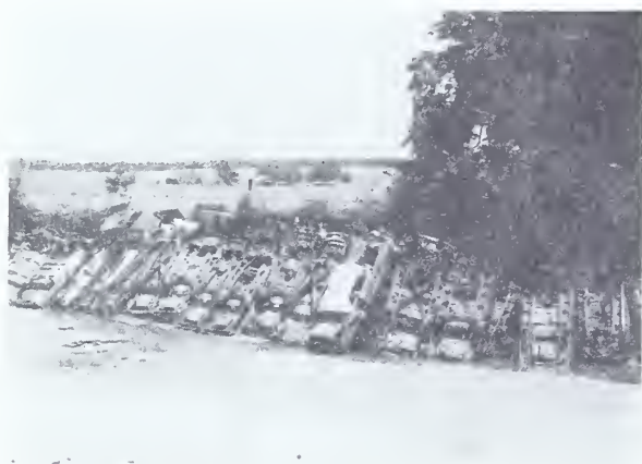
Figure 9.--Upstream end of bank protection placed on Winter Creek north of Alex, Okla.
