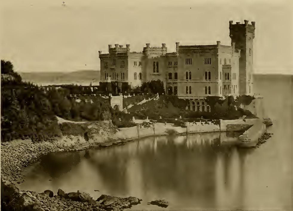
VIEW OF MIRAMAR
