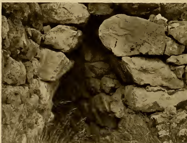
ANCIENT ARCH CONSTRUCTION, MYKENÆ
