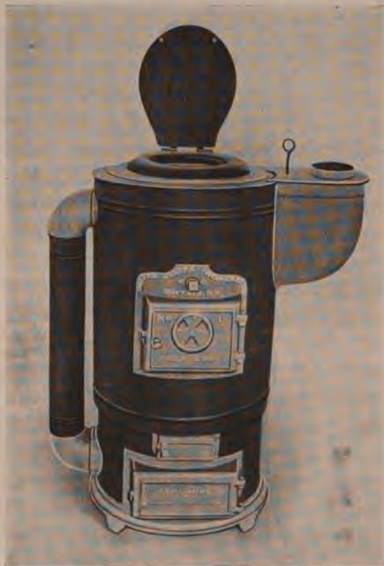
Fig. 36.—Incinerator for excreta; United States Incinerator Co. type.
