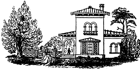
[Fig. 65. Gate Lodge in the Italian style.]
