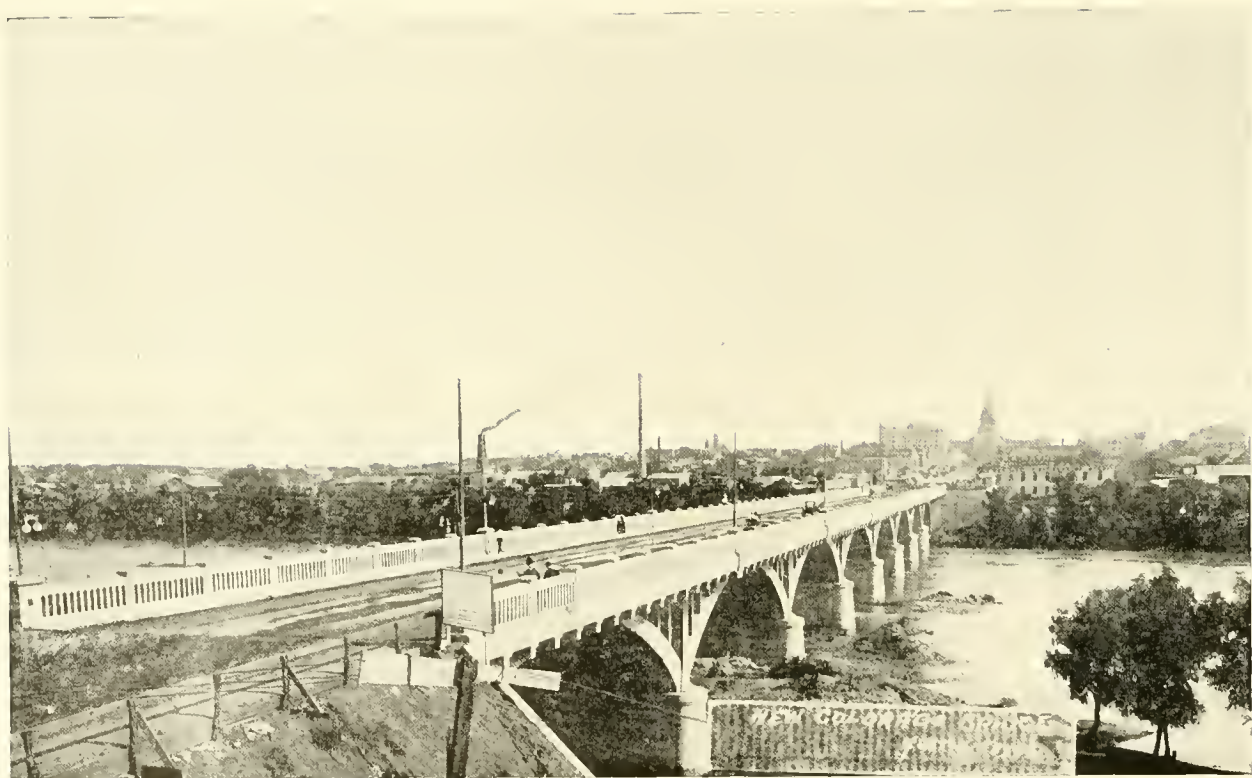
THE BRIDGE—CROSSING THE COLORADO AT AUSTIN.
