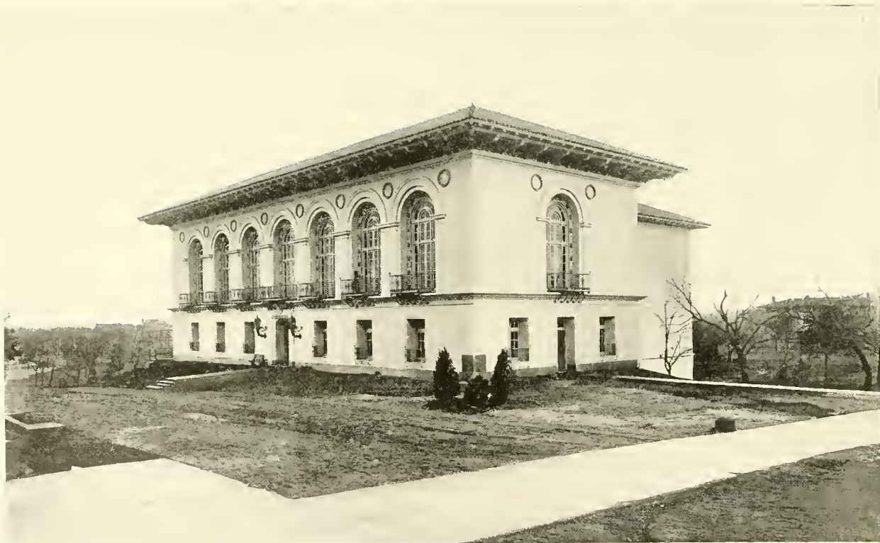
THE UNIVERSITY LIBRARY—ONE OF THE BEST PIECES OF ARCHITECTURE IN TEXAS.
