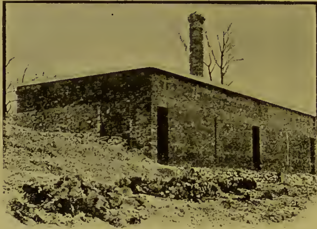
FIG 28. FILTER HOUSE AT CATERHAM.
