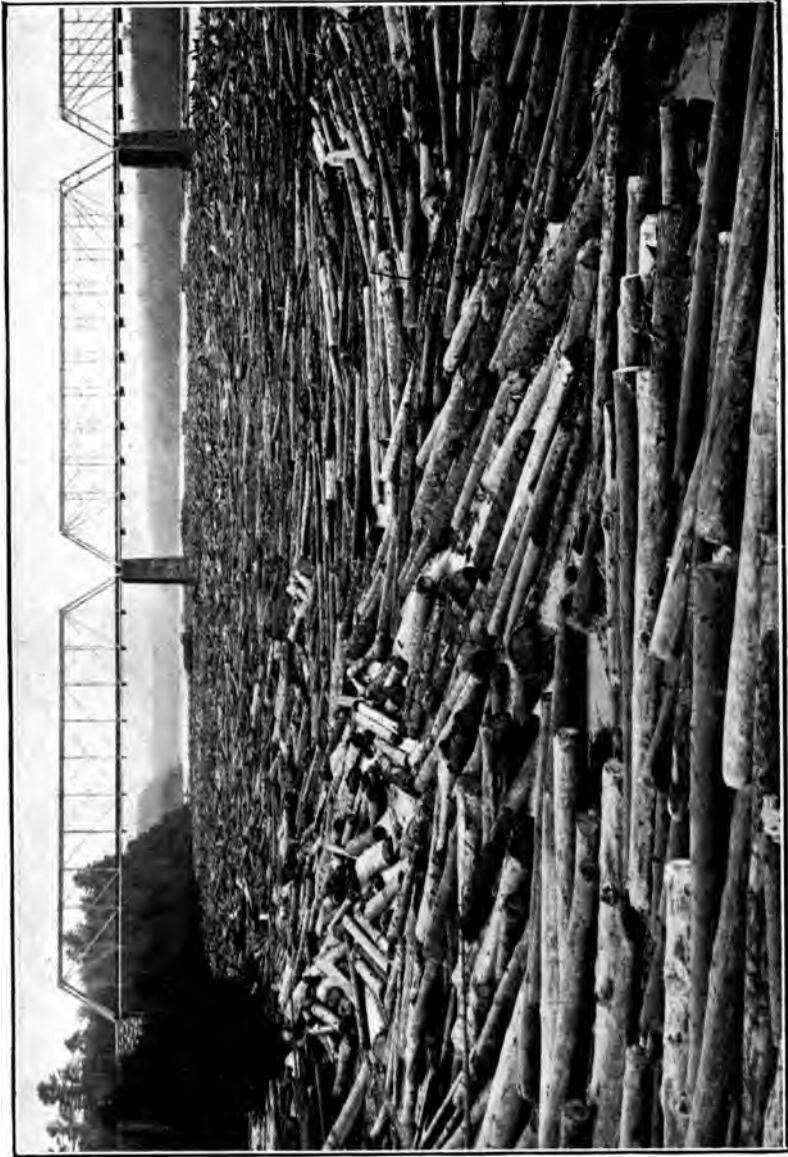
LOGS AT CANADIAN PACIFIC RY. BRIDGE, AT THREE RIVERS, P.Q.
