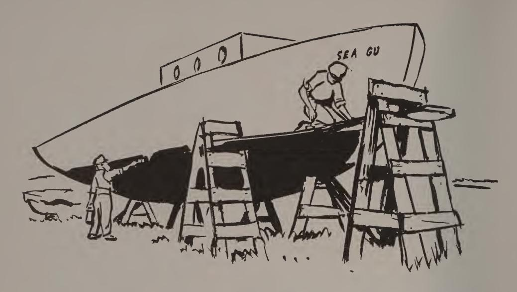
The painters began painting the hull. The part below the water was red. The topsides above the water were white. The deck was green. The cabin was varnished. Four coats of paint were spread on to make the boat waterproof and preserve the wood. The boat's name SEA GULL was painted on the side. Everyone said the boat was beautiful. Sailmakers had made sails for the boat.
