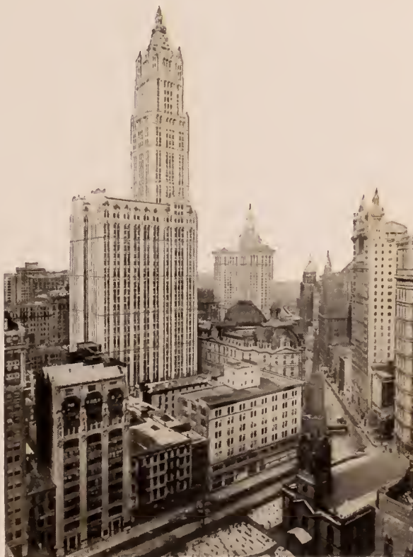
VIEW FROM THE SOUTHWEST
