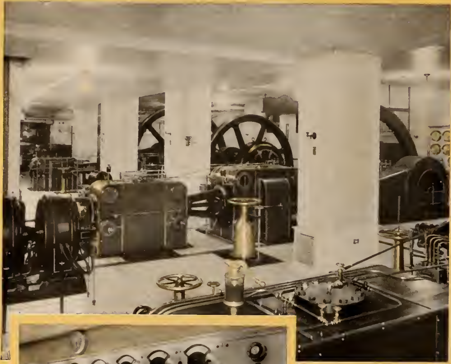
GENERATORS AND MAIN SWITCHBOARD IN THE ENGINE ROOM
