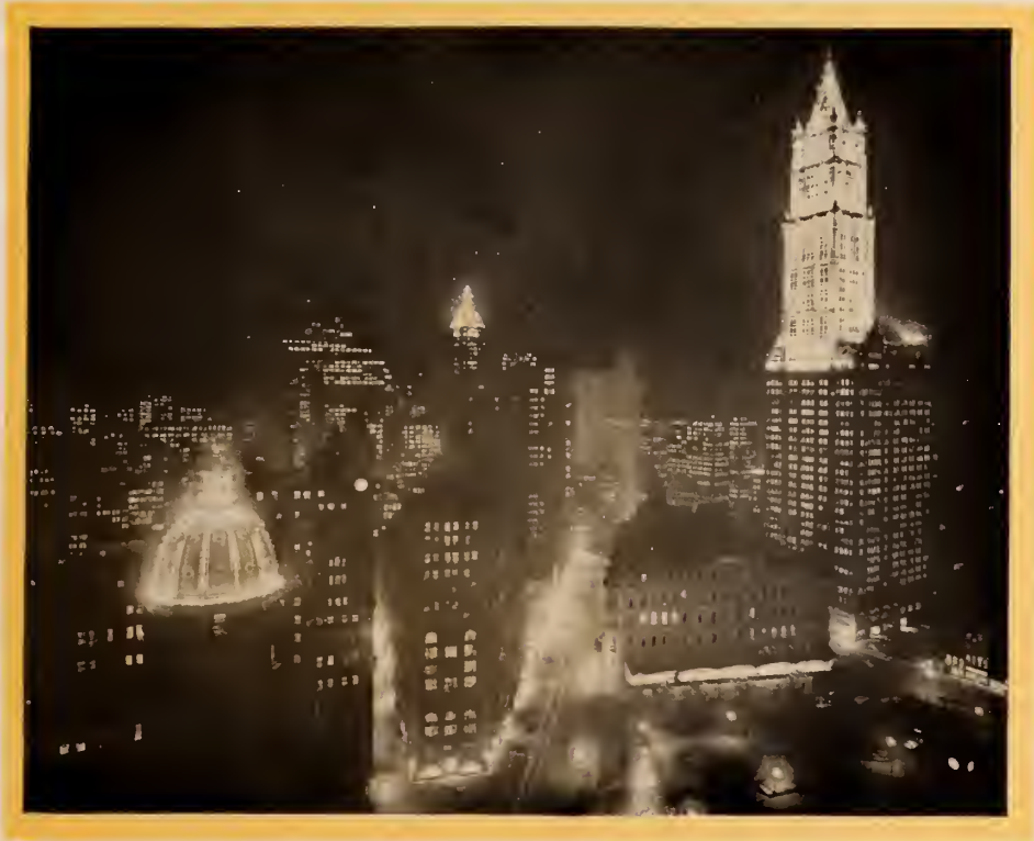
THREE TOWERS OF LOWER MANHATTAN AT NIGHT
