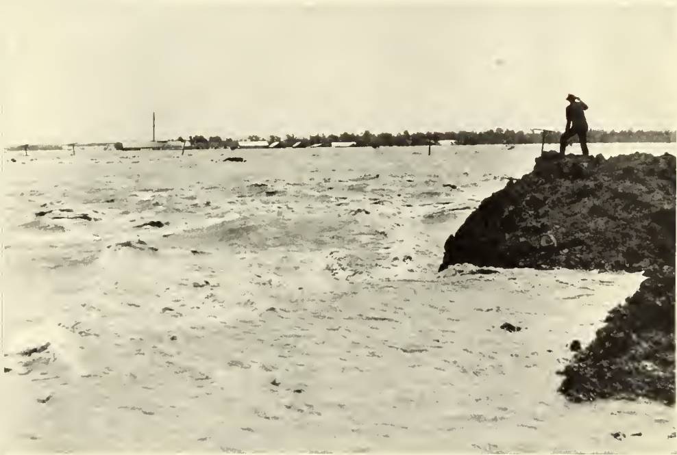
LIKE A CATARACT, FLOODS RACE THROUGH CRUMBLING LEVEES
