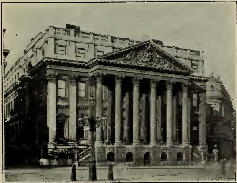
Fig. 7. Mansion House, London.
