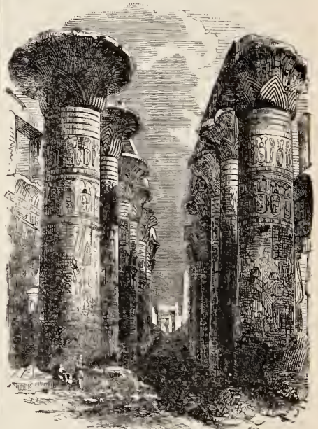
Temple at Karnak (Thebes). Columns in the great Hall. (From a Photograph.)
