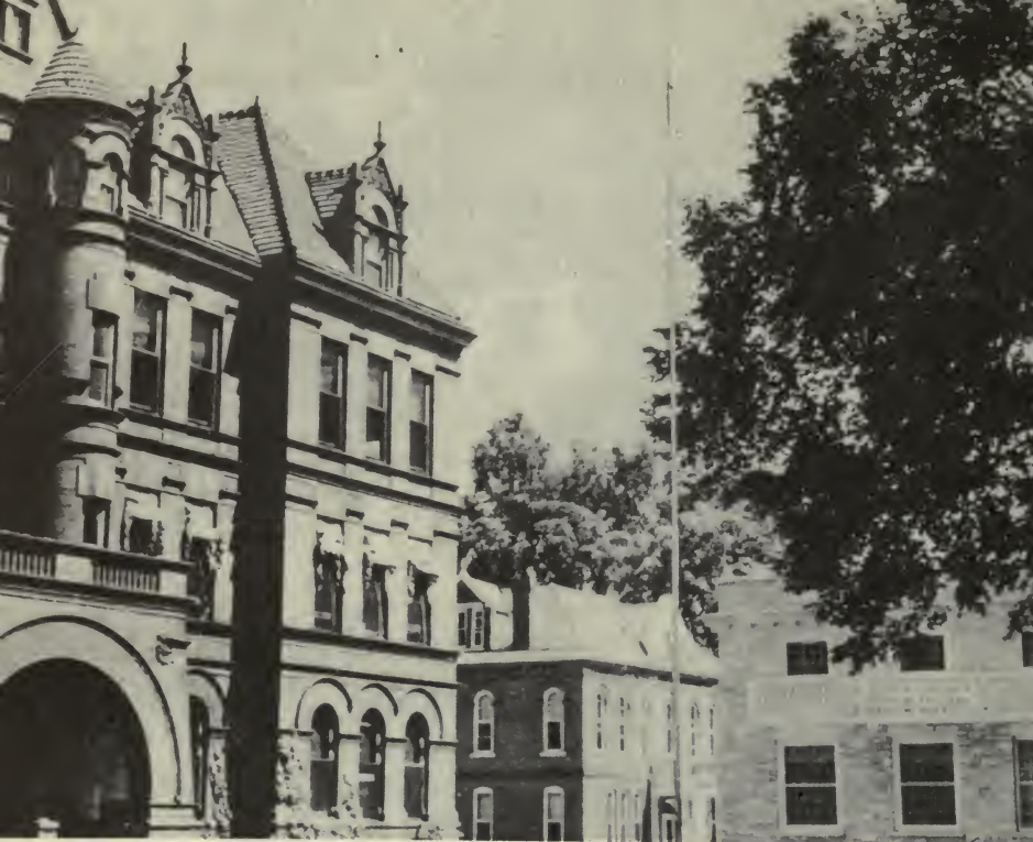
County Seat, Wheaton: Old Courthouse, Sheriff's House, New Courthouse
