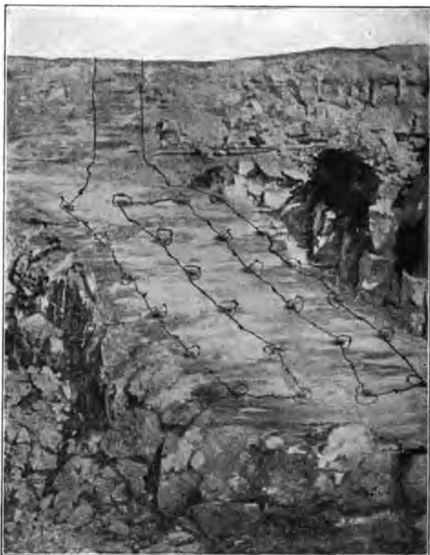
Twenty-four holes with two electric blasting caps in each hole—48 electric blasting caps in all—connected in series. The blast should be fired with a No. 4 or a No. 5 Du Pont Blasting Machine, or with a power or lighting circuit of 110 volts and 1\frac{1}{2} amperes.
