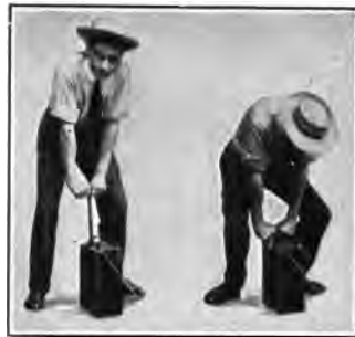
OPERATING A DU PONT BLASTING MACHINE
