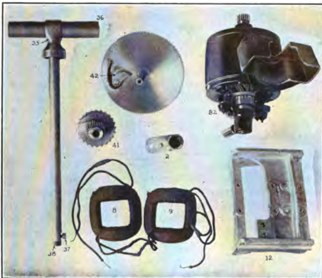
PARTS OF DU PONT No. 6 BLASTING MACHINE
