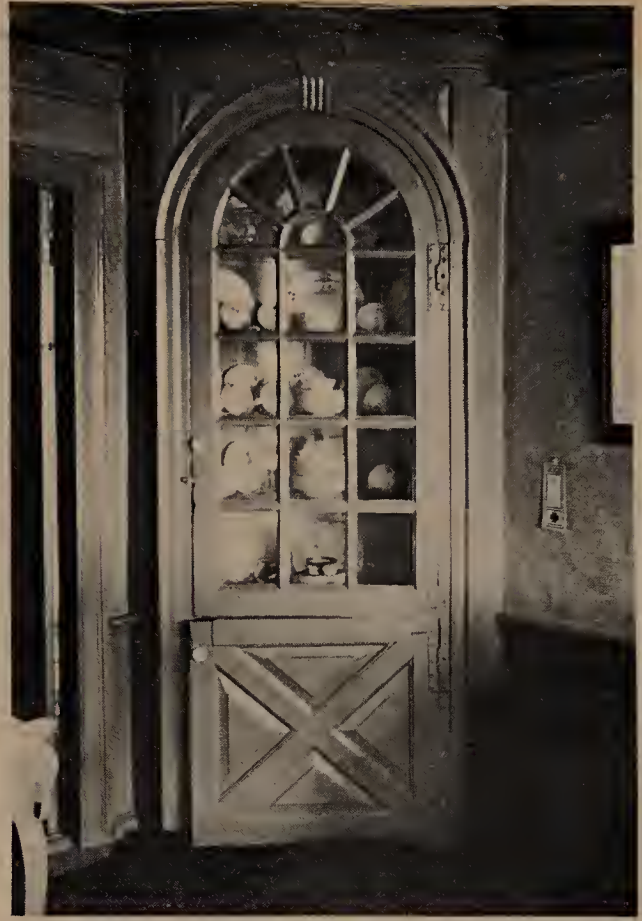
CUPBOARD IN AN OLD HOUSE— WEST HARTFORD
