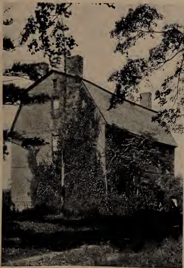
BRADLEY HOUSE—NORTH HAVEN
