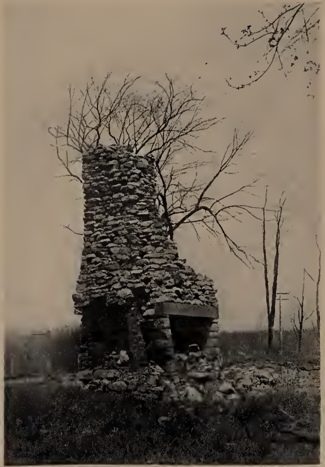
CHIMNEY OF A COLLAPSED HOUSE— CHESHIRE
