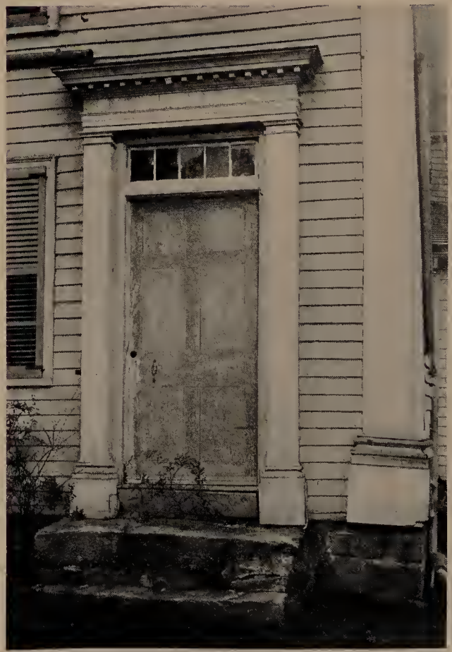
ELY HOUSE—ELY'S LANDING
