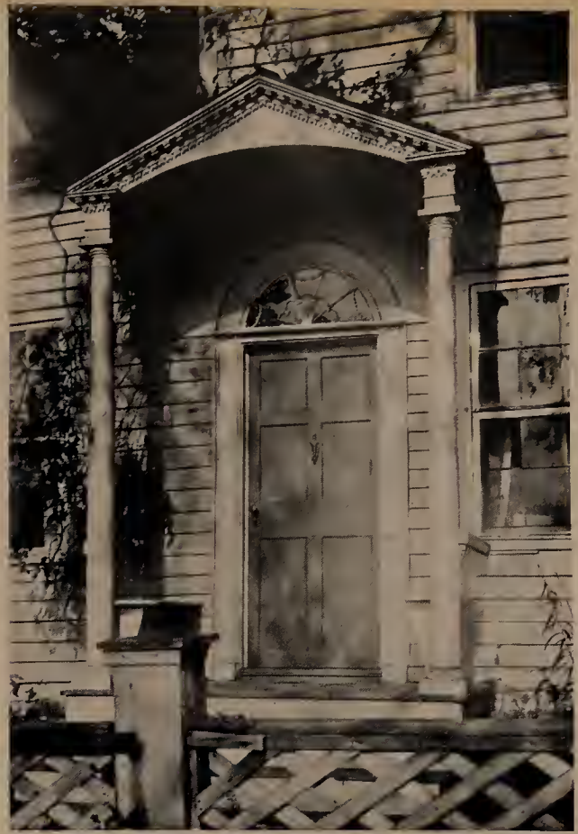
ENTRANCE OF AN OLD HOUSE— REDDING RIDGE
