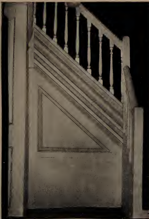
GENERAL JOHNSON HOUSE—GUILFORD
