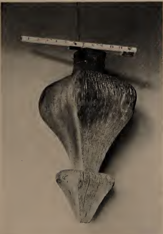
FROM A DEMOLISHED HOUSE—FARMINGTON
