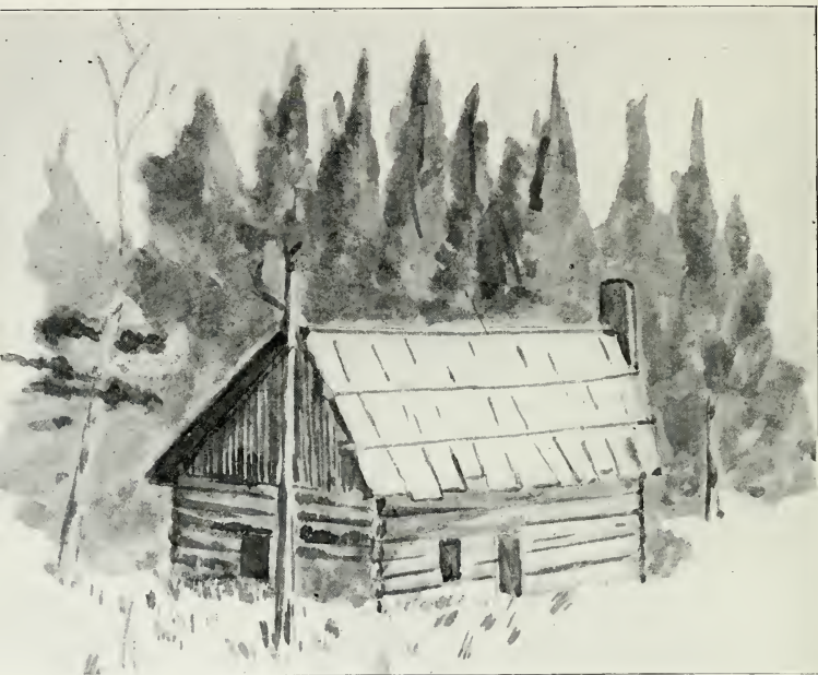
THE FIRST LOG CABIN Built in the Maumee Valley, near Fort Miami,
