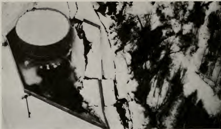
A close-up of the compressional buckle, the ruptured fuel tank, and the revetment at the foot of the landslide near the Alaska Native Hospital, Anchorage.
