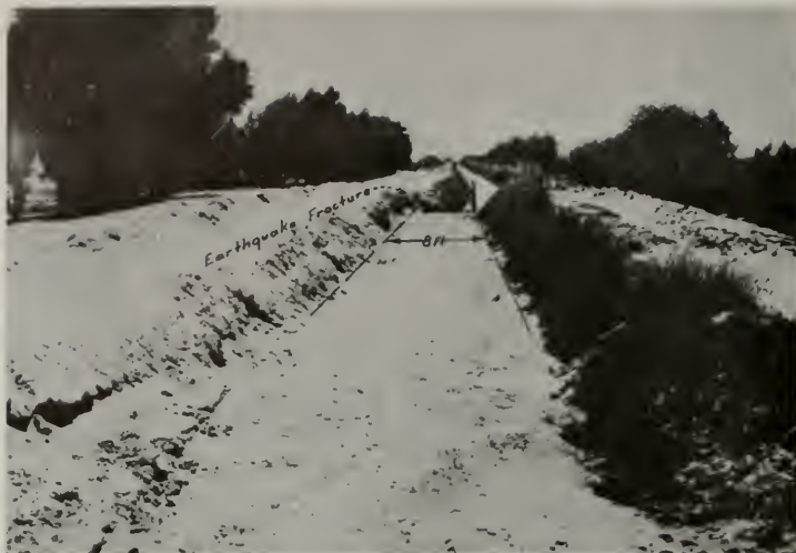
Canal Offset by Imperial Fault Imperial Valley Earthquake, May 18, 1940
