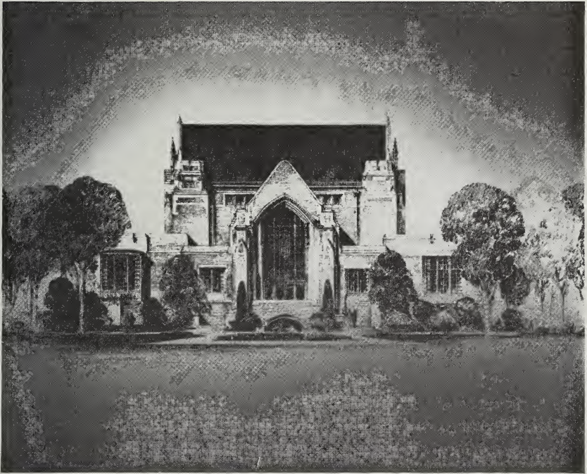
THE MARY J. BOOTH LIBRARY Under construction, 1949
