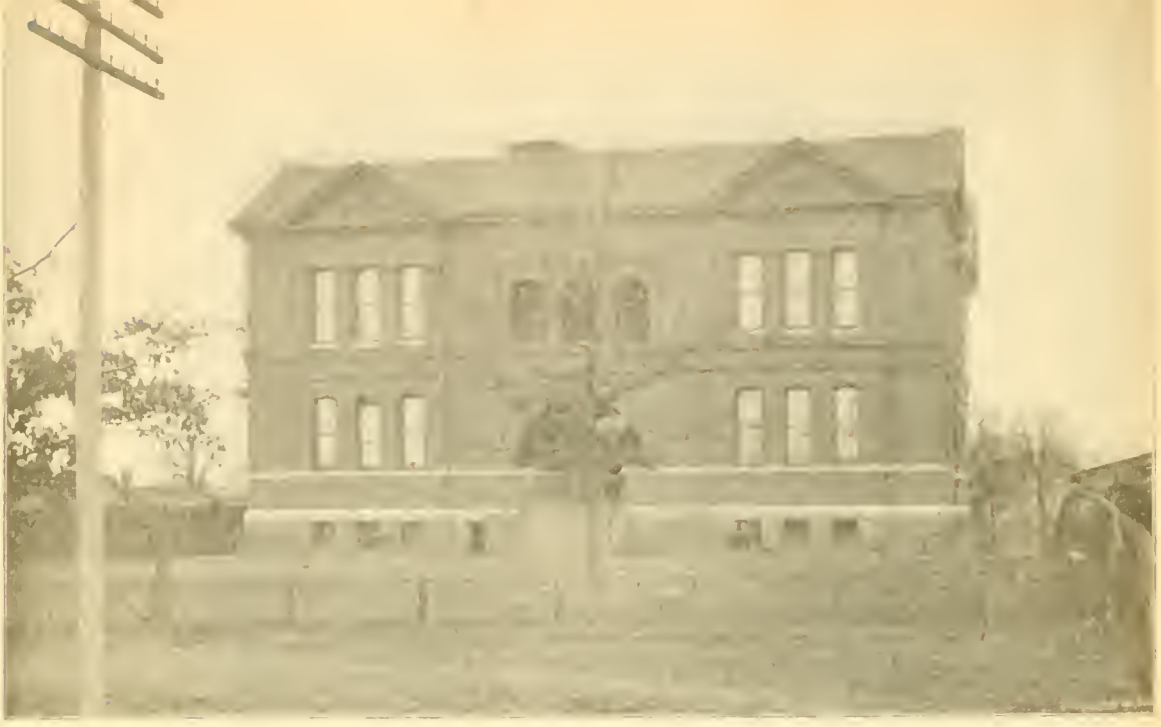
EDGEWOOD AVE. PUBLIC HIGH SCHOOL, ATLANTA, GA.
