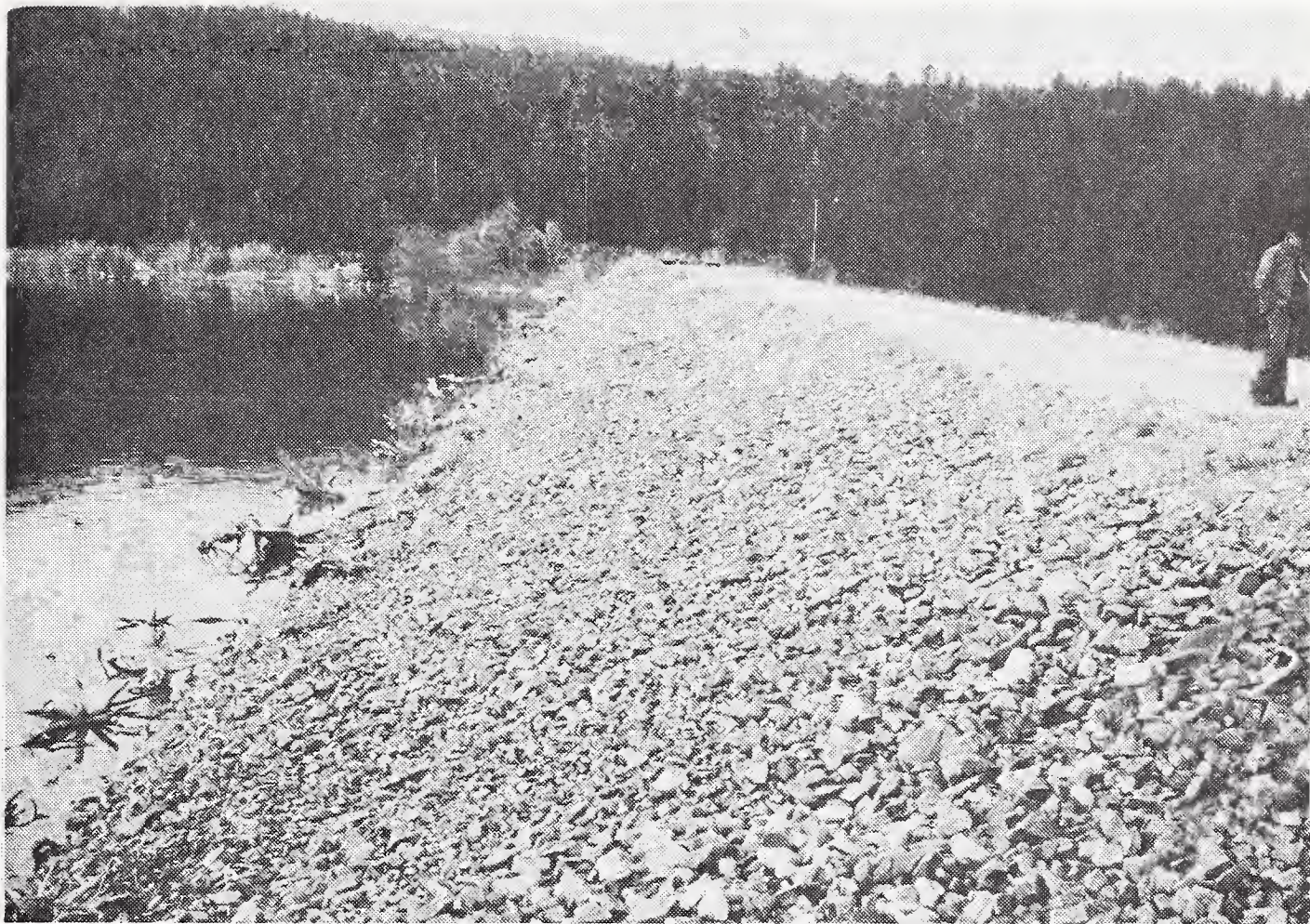
(PHOTO 3) Embankment Upstream Slope.
