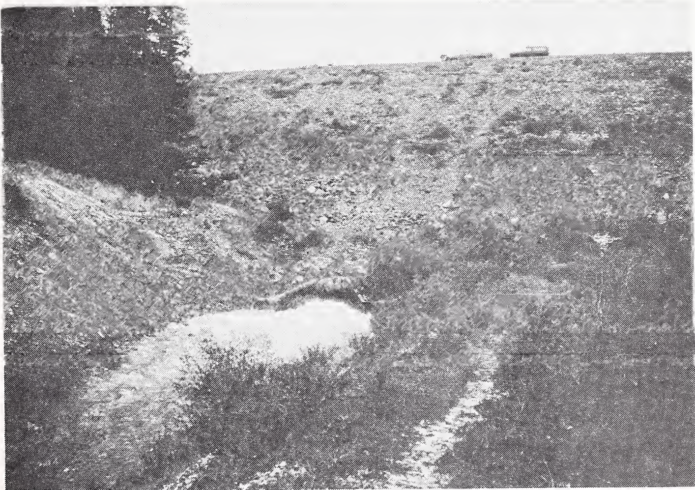
(PHOTO 2) Outlet channel and Right abutment .
