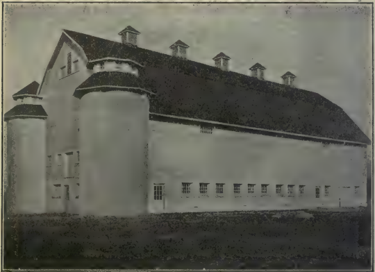
85. Cement silos and stock barn
