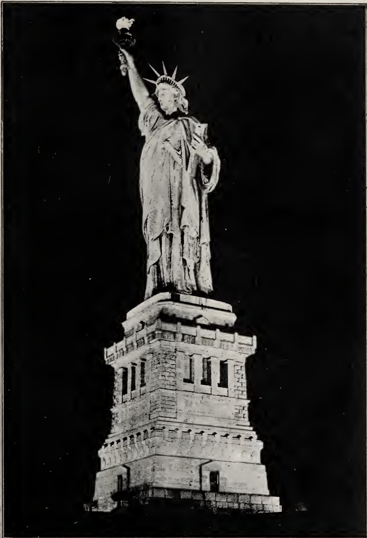
FIG. 334. — Statue of Liberty illuminated at night by means of 15 batteries of flood-lighting projectors using 250-watt tungsten lamps.
