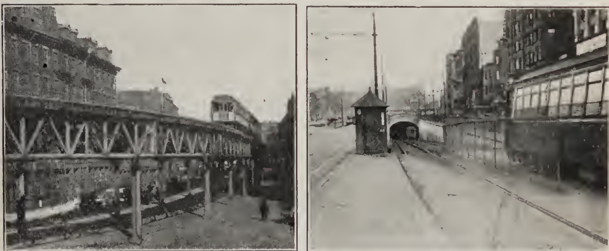
FIG. 359. — City streets showing elevated structure and entrance to subway.
