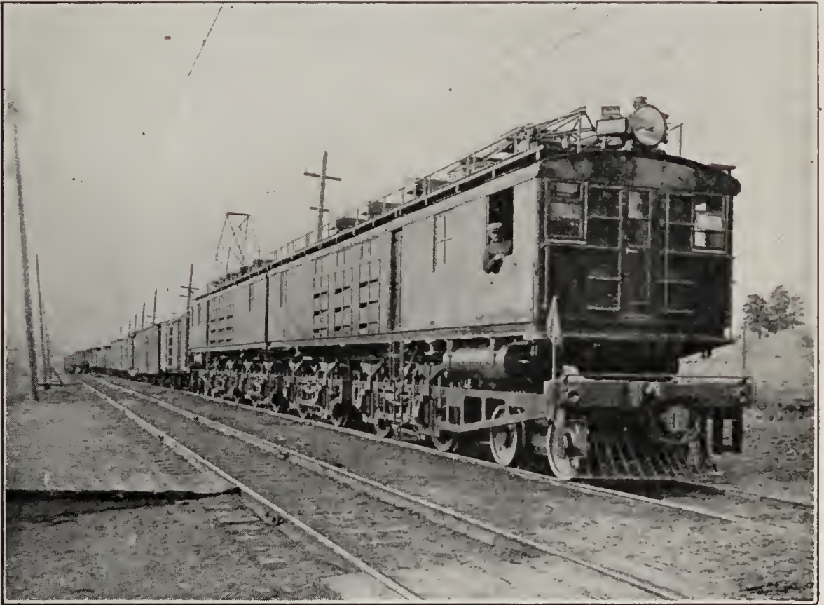
FIG. 363. — Electric freight locomotive used on C. M. & St. P. Ry. hauling a freight train of 40 cars, 1640 tons.
