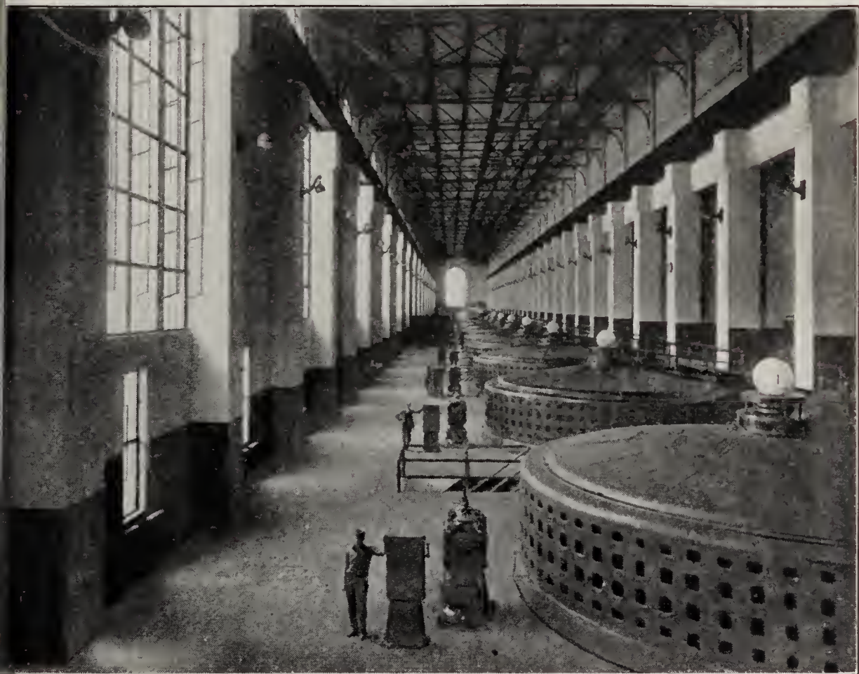
FIG. 291. — Mississippi River Power Company (largest in the world) with fifteen 9000-kv-a. 11,000-volt generators. The ultimate installation will have double its present capacity.
