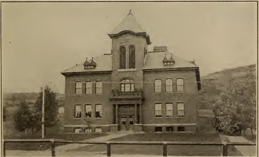
Illus. 14. Entire Basement Floor of This School and Walk 10 ft. by 90 ft. Laid by Eighth Grade Boys.
