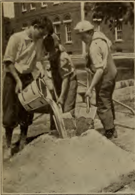
Illus. 4. Applying Water to Mixture.
