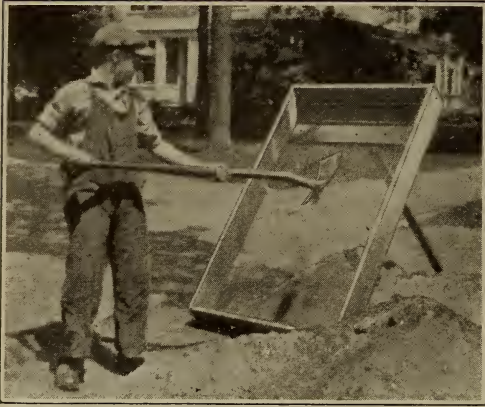
Illus. 2. Sifting Sand Before Mixing.
