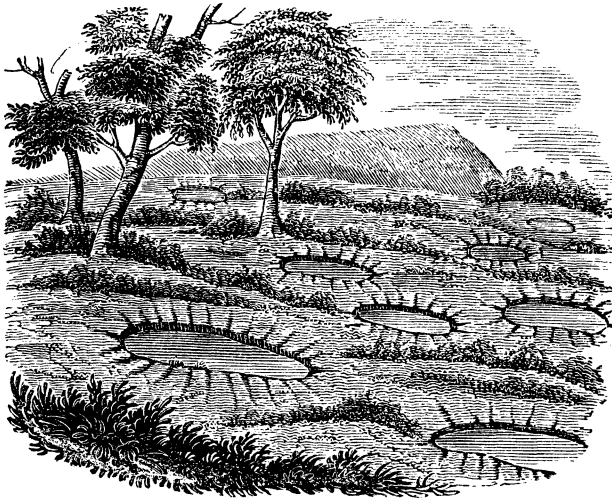
Holes formed by an Earthquake.
