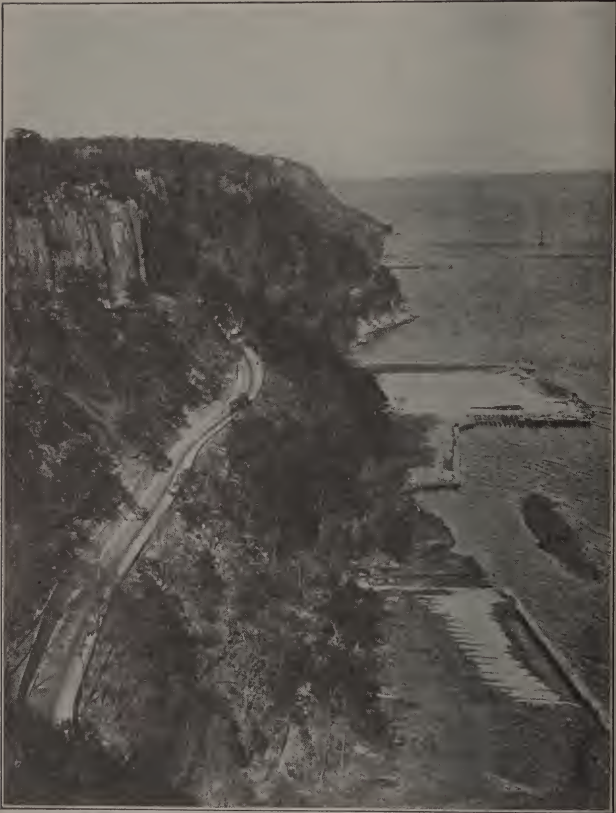
A MODERN WAY TO CLIMB THE PALISADES.
