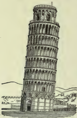
FIG. 23.—The Leaning Tower of Pisa. It overhangs its base more than 13 feet, but it is stable. (Drawn from a photograph.)
