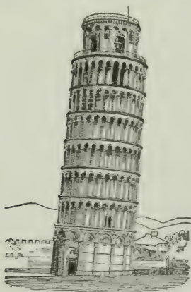
FIG. 23.—The Leaning Tower of Pisa. It overhangs its base more than 13 feet, but it is stable. (Drawn from a photograph.)
