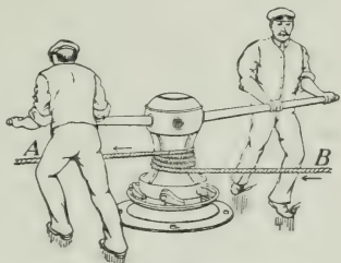
FIG. 50.—Raising the ship's anchor by a capstan.
