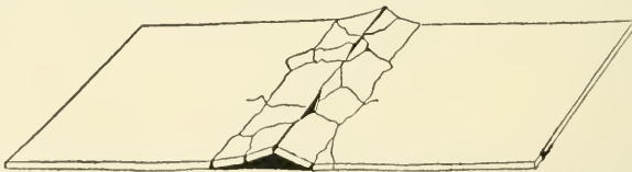
Fig. 17.— A cement walk broken under expansion by sun-heat.
