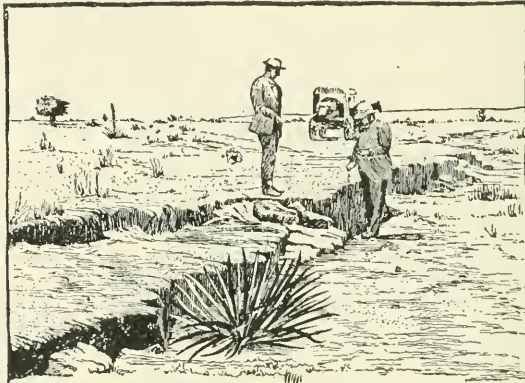
Fig. 198.—Fissure produced by earthquake. Arizona.
