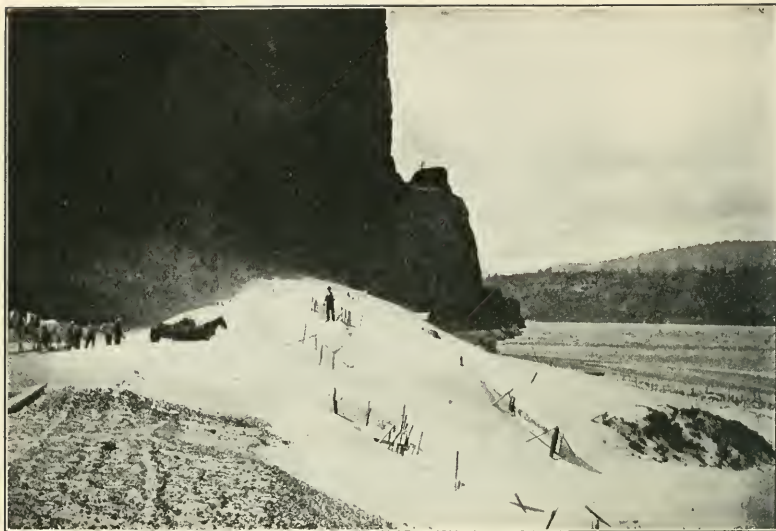
Fig. 1.—Sand drifted over a railway. One rail shows at the left-hand side. Rowena, Wash. (U. S. Dept. of Agr.)
