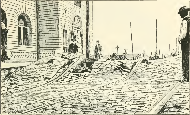
Fig. 195.—Deformed railway, Seventh and Mission Streets, San Francisco.
