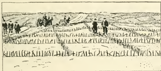
Fig. 14.— Dune sand held by brush fences on the Kurische Nehrung.
