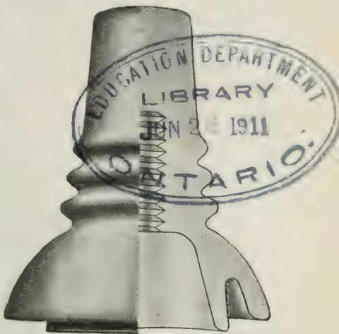
FIG. 100.—Langdon insulator.
