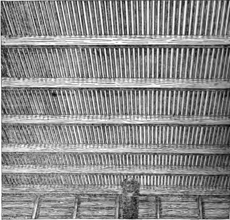
FIG. 21.—Detail of the floor construction of a hop-kiln drier, from below.
