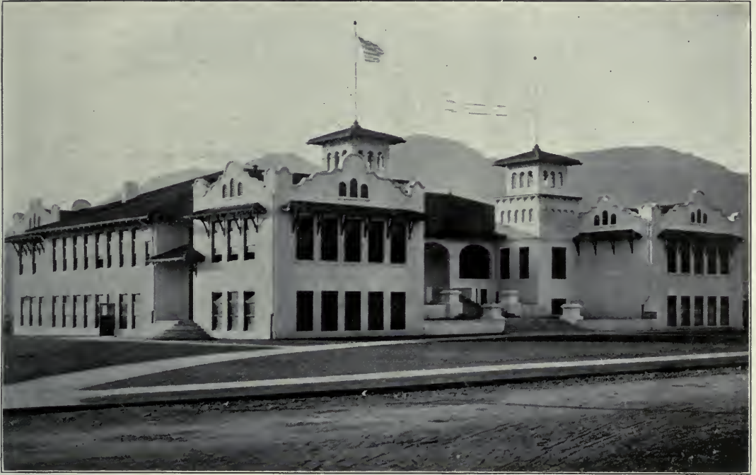
FILLMORE UNION HIGH SCHOOL, FILLMORE, CAL. A. C. Smith, Architect, Los Angeles, Cal.
