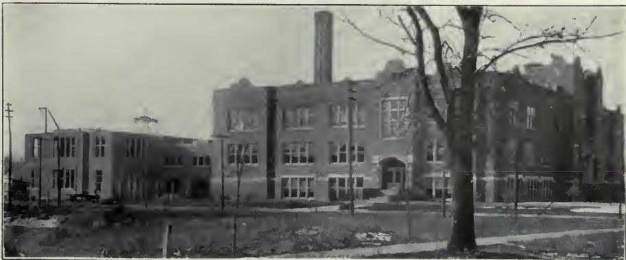
SIDE VIEW, LA CROSSE HIGH SCHOOL (Manual Training Addition under Construction)
