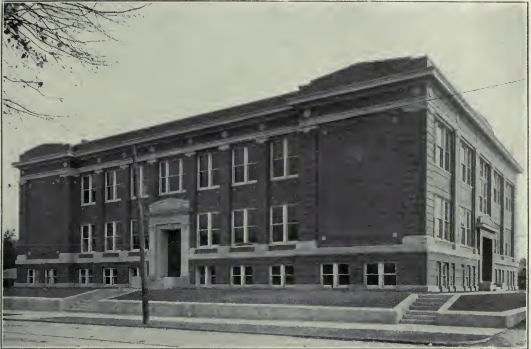
HIGH SCHOOL, LEBANON, IND. Herbert L. Bass & Co., Architects, Indianapolis, Ind.
