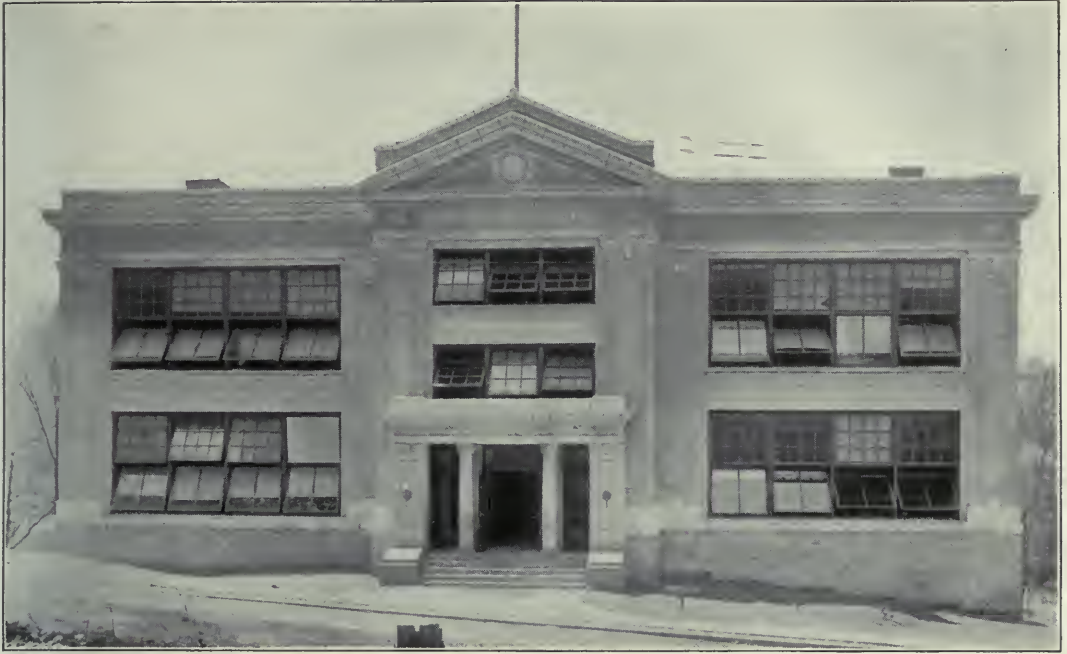
HIGH SCHOOL, WOODLAWN, PA. C. C. & A. L. Thayer, Architects, New Castle, Pa.
