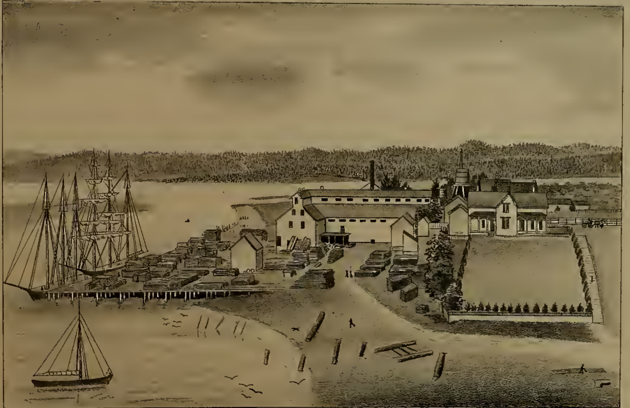
"BAY MILL" & RESIDENCE OF DOLBEER & CARSON, EUREKA, CAL. CONSTRUCTED, 1878. CUTTING CAPACITY, PER DAY, 60,000. " " " YEAR 9,580,000. " " SHINGLE - 2,800,000.
