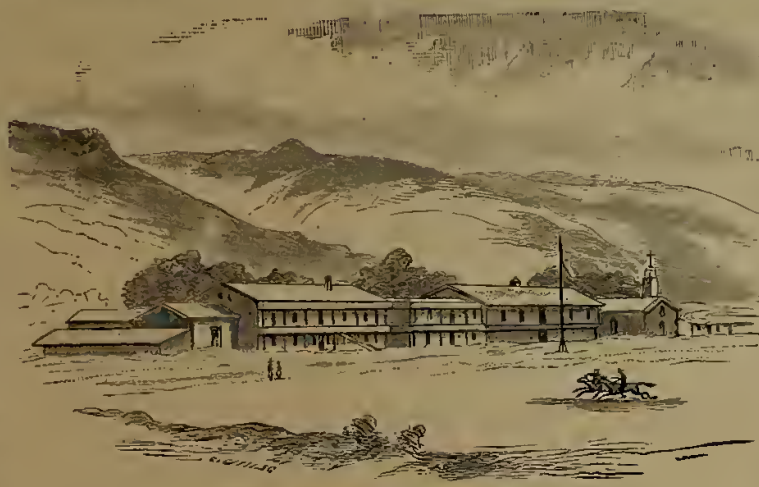
MISSION CHURCH AND BUILDINGS AT SONOMA.
