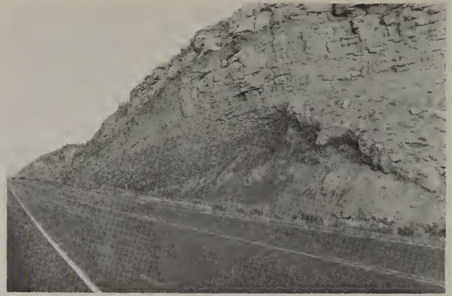
Figure 4. Outcrop of the Washboard unit of Cotter (1975a) of the Ferron Sandstone Member of the Mancos Shale along U.S. Highway 6 southeast of Wellington. View facing northwest.
