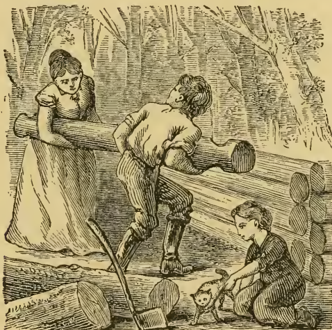
BUILDING THE CABIN-HOME.
