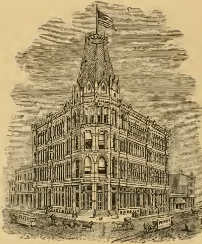
VANCE BLOCK, INDIANAPOLIS.
