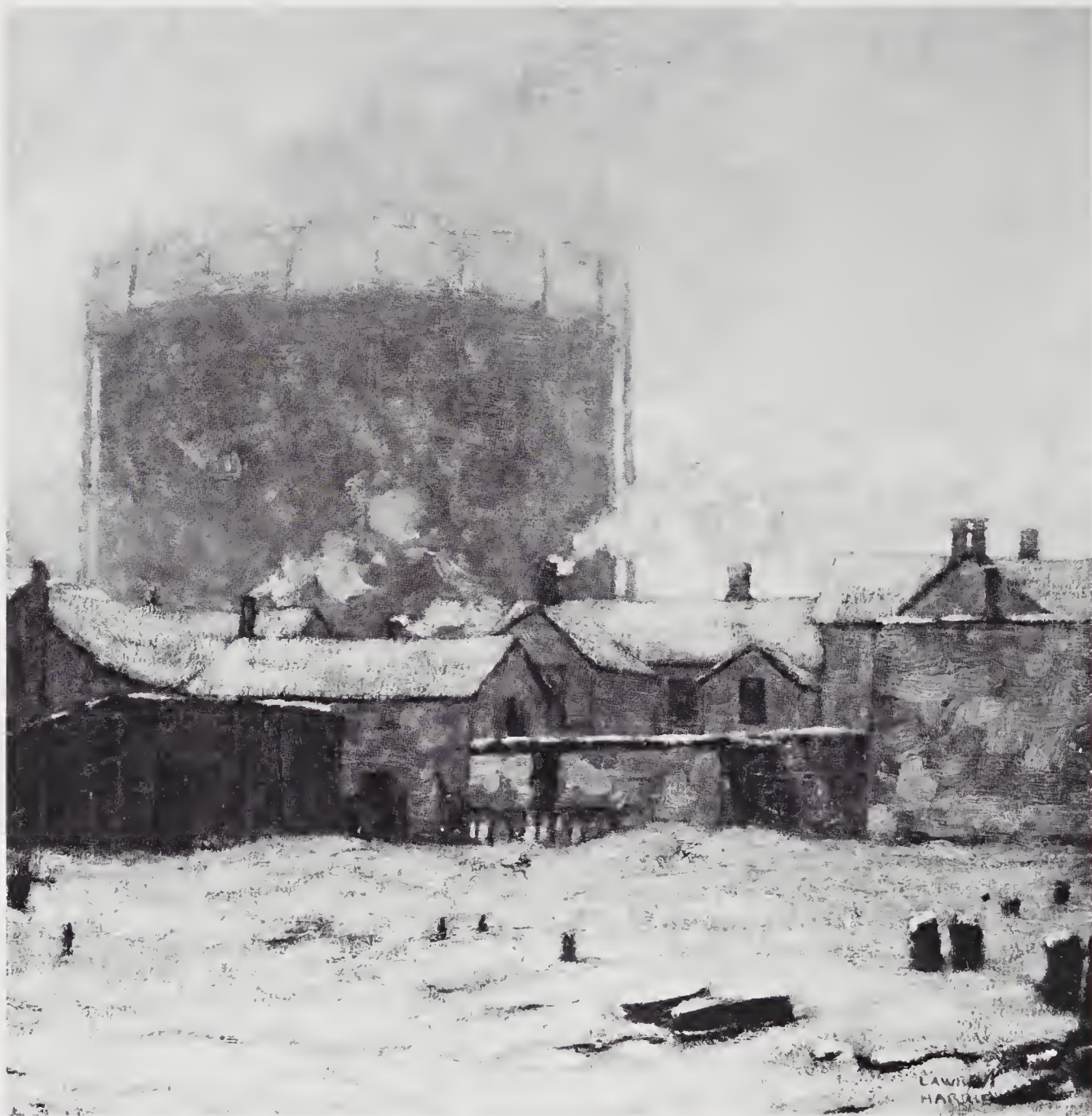
21. The Gas Works, 1911-12
